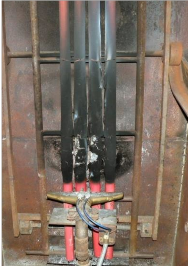
Figure 2 – Fire test according to IEC 60332-3 (source TB 720)
