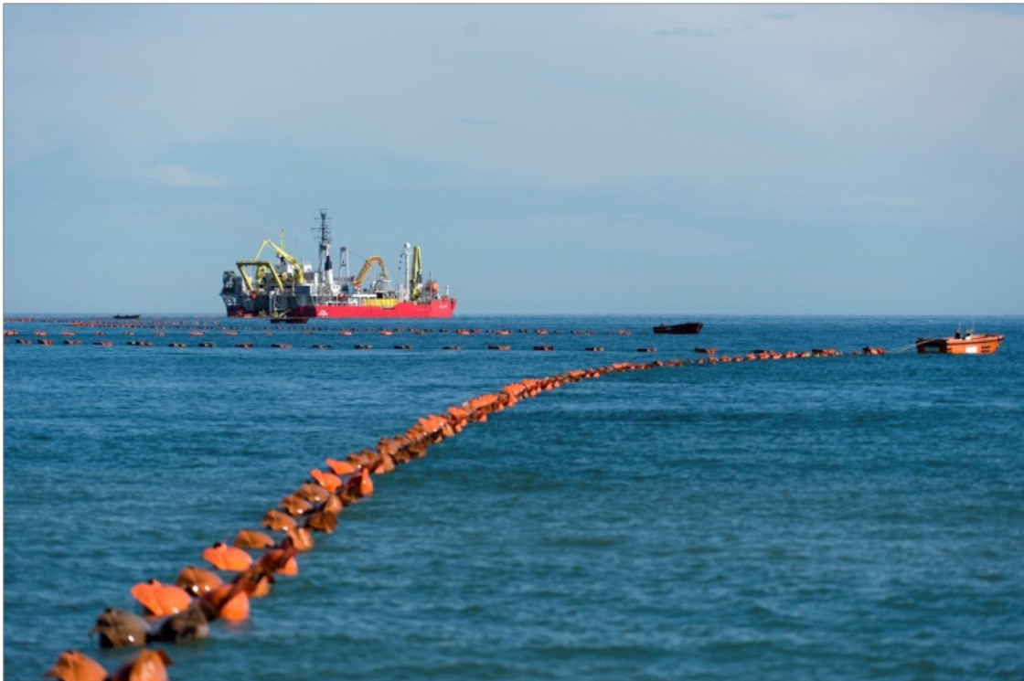
Figure 1 – Laying activities for Submarine cables (source TB 610 )
