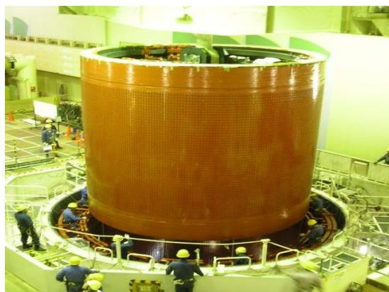
Photograph: Rotor of 400 MW, 330-390 min-1, 700 tons, 6000 mm, asynchronous generator-motor
