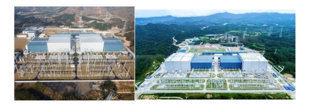
(a) Liubei station (3000MW) (b) Longmen station (5000MW) Figure 2 - Images of the ±800kV VSC convertor station
