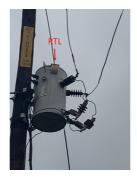
Figure 2 - An RTL installed on a transformer tank
