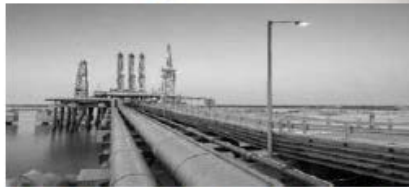
Aqaba Terminal Infrastructure
