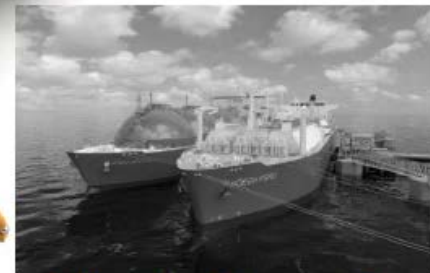
Floating Storage & Regasification Unit
