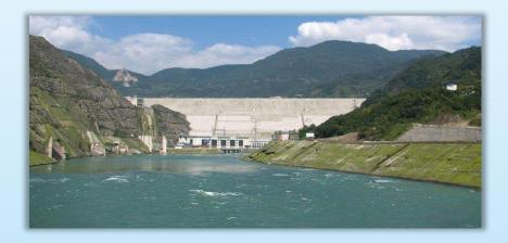
Located at the upper reach of Min River in Northwest Chengdu, Sichuan Province, (9km away from Dujiangyan City), Zipingpu Hydropower Station is a large hydraulic project primarily for irrigation and water supply with a combination of power generation, flood prevention and sightseeing functions. It has an installed capacity of 760MW, an annual power generation of 3.417TWh and an annual utilization hours of 4496h.
